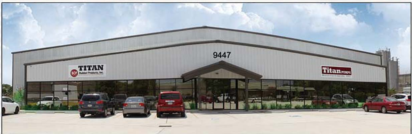
Titan Manufacturing Facility: 45,000 sq. ft.
